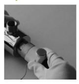
Step 11: Insert the earth cable tightly.
